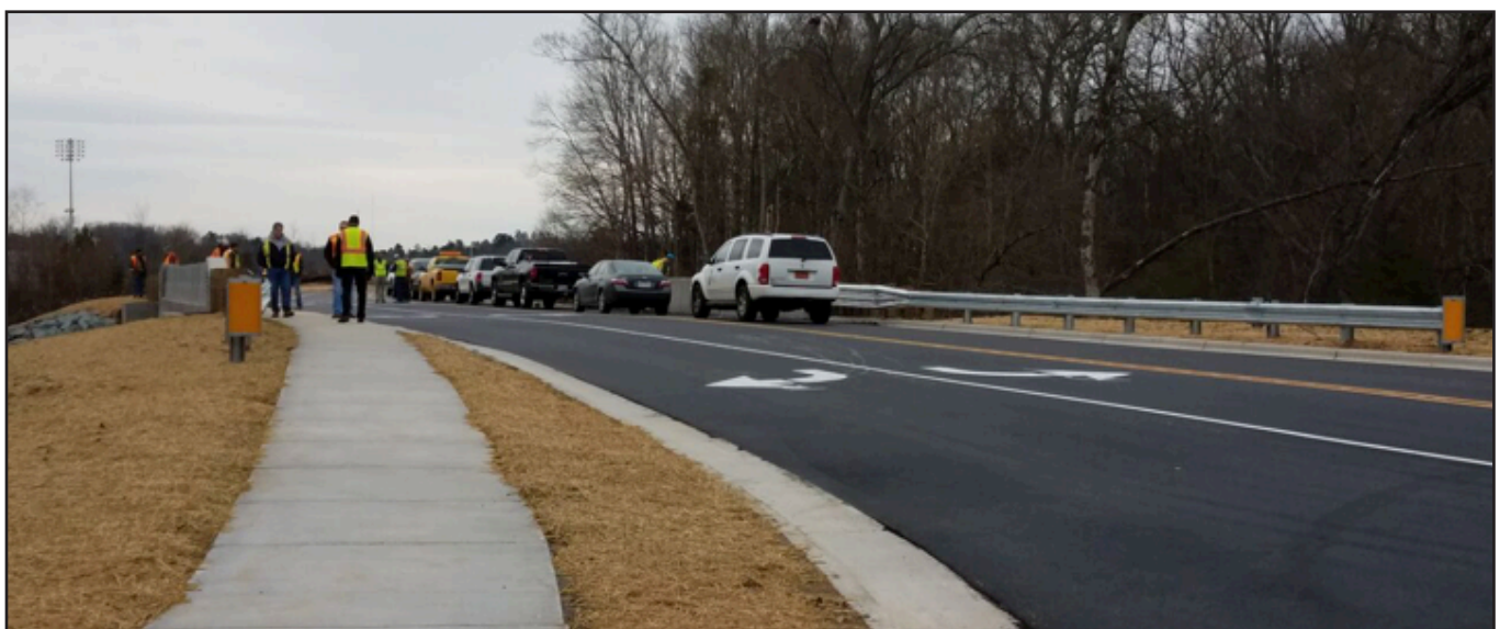
Bridge replacement project with new sidewalk- Raging Ridge Road at Stallings Road in Harrisburg.
